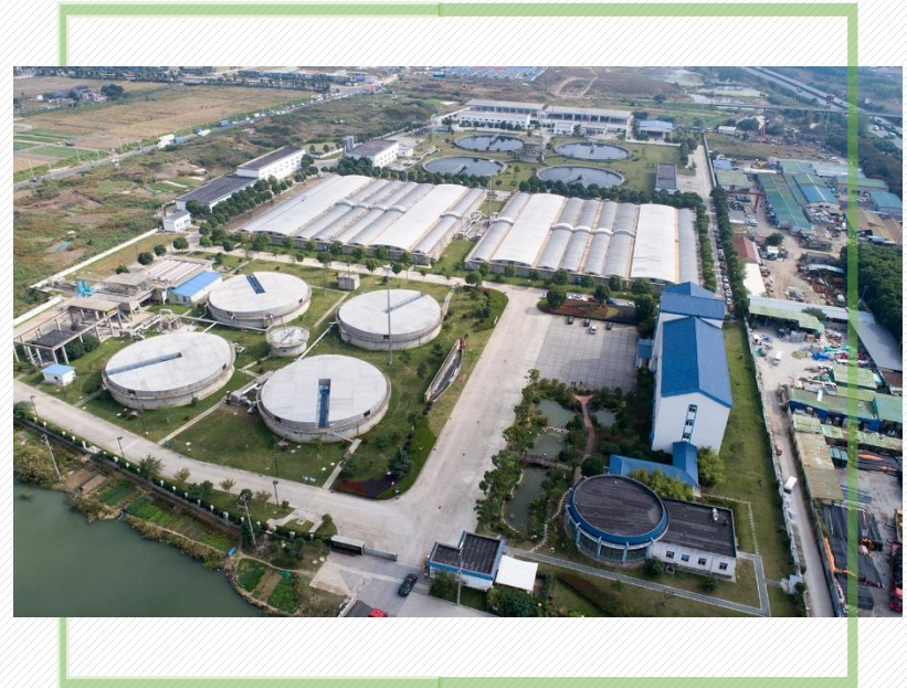
Suzhou Wuzhong Chengnan WWT Plant
