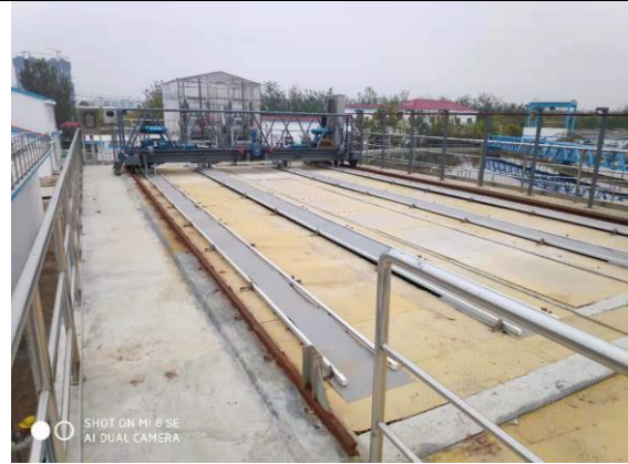
曝气沉砂池封盖
